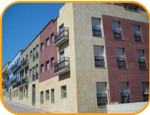
LATERAL VIEW OF THE 30 FLAT BUILDING
